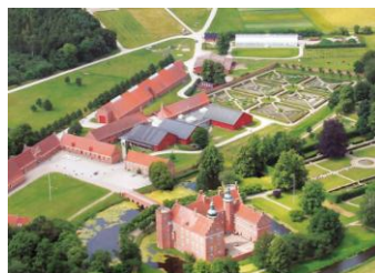
Figure 11. The Green Museum, Denmark
